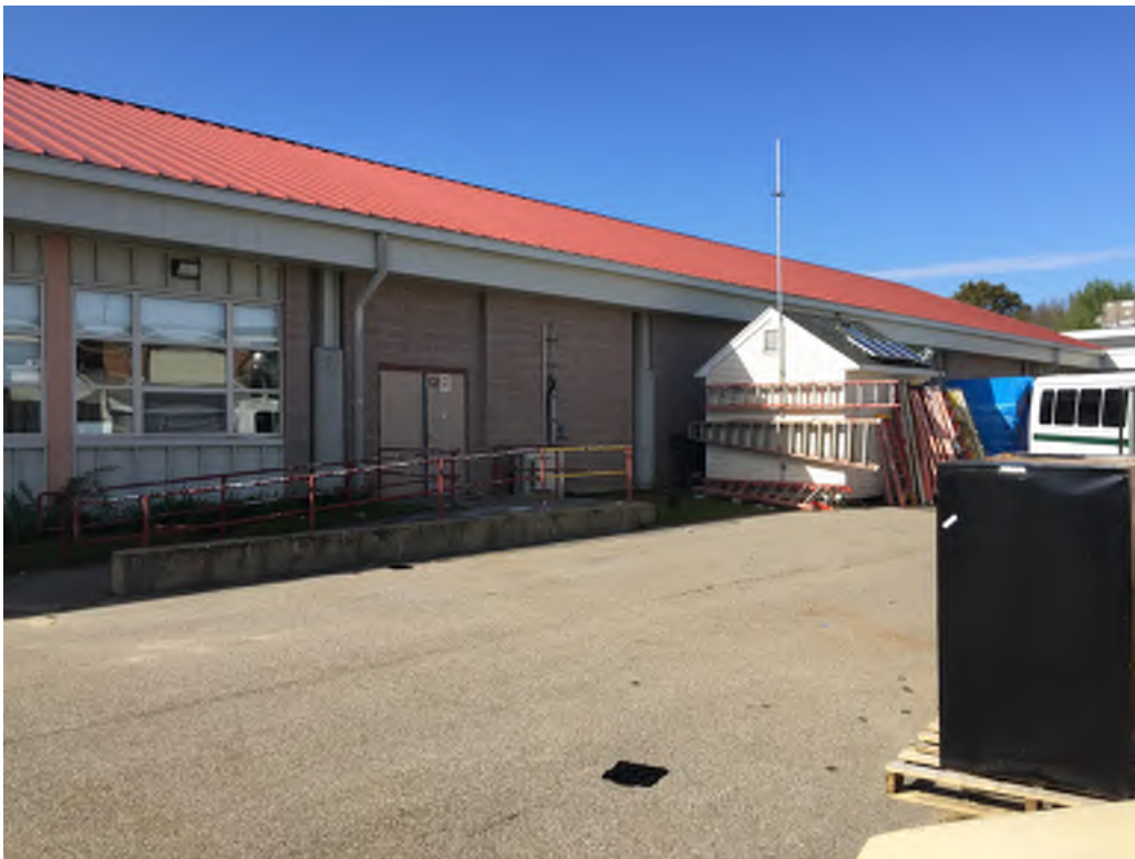
Photograph of the 1992 Addition looking towards the Electrical Shop
