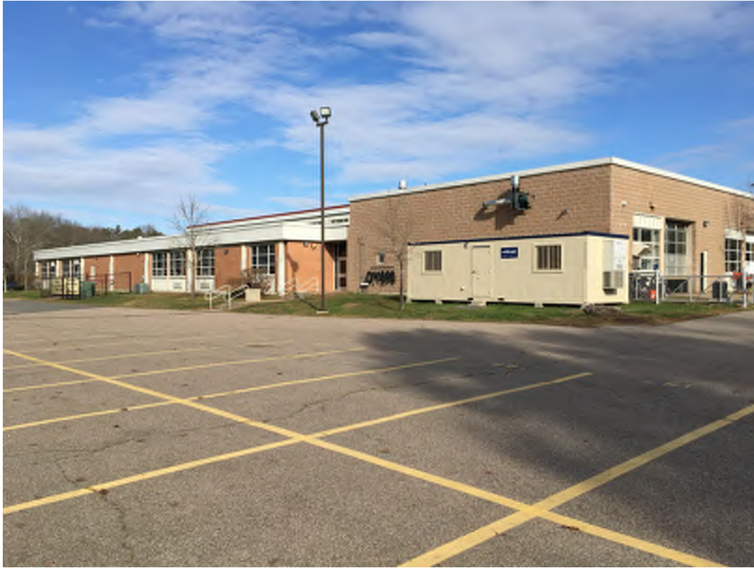
Photograph of the 1992 Addition looking at Auto Collision
