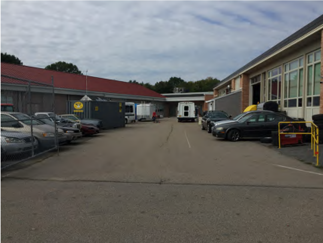
Photograph of the back courtyard in the 1992 Addition
