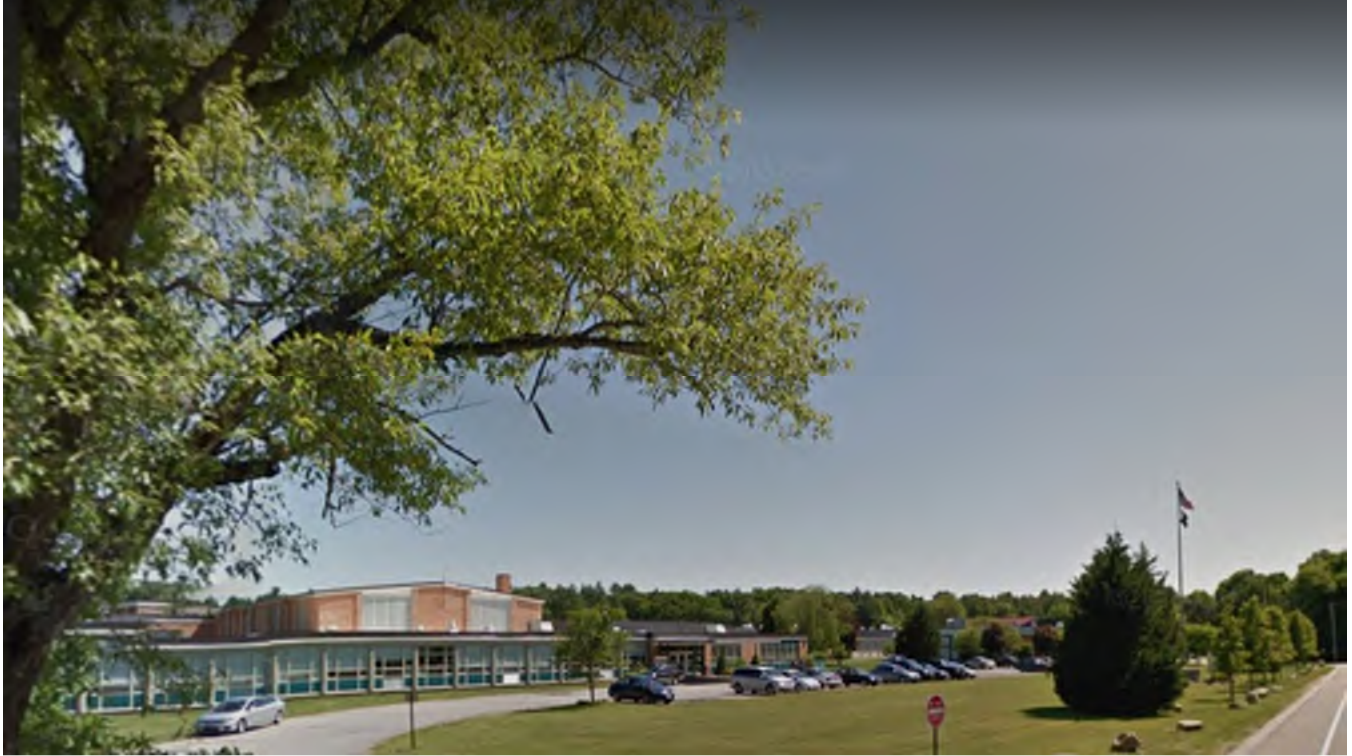
Front Façade View along Webster Street
