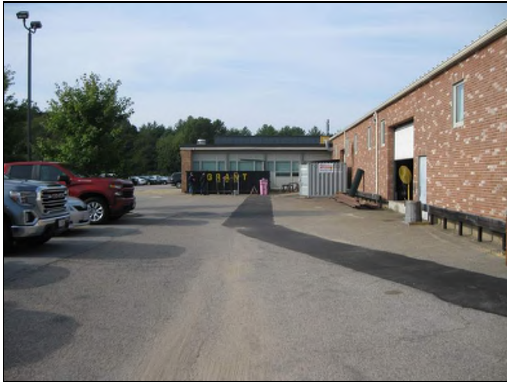
Southeast side of school
