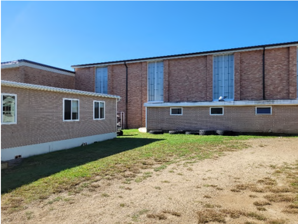
Figure 5: Typical Roof Leaders Connecting to Closed Drainage System
