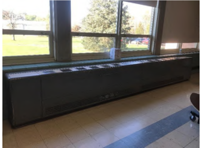
M6 - Typical hydronic radiation
