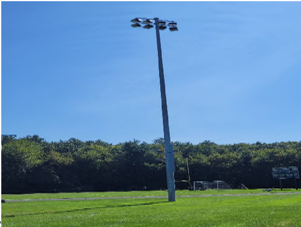
Figure 7: Light Pole at the Athletic Field
