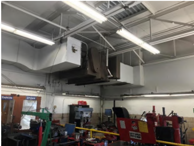
M11 - Typical ducted fan coil unit.
