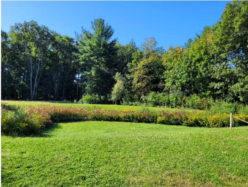
Figure 5: Stormwater Detention Basin
