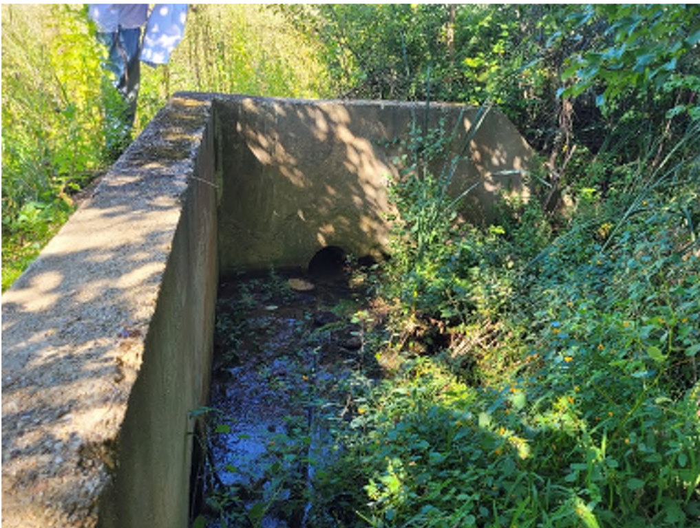
Figure 4: Concrete Headway for 18-Inch and 30-Inch Outlet Pipes
