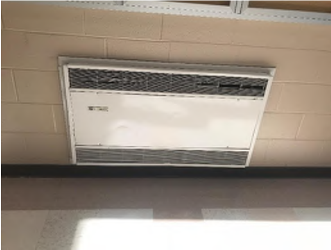
M5: Typical hydronic cabinet unit heater
