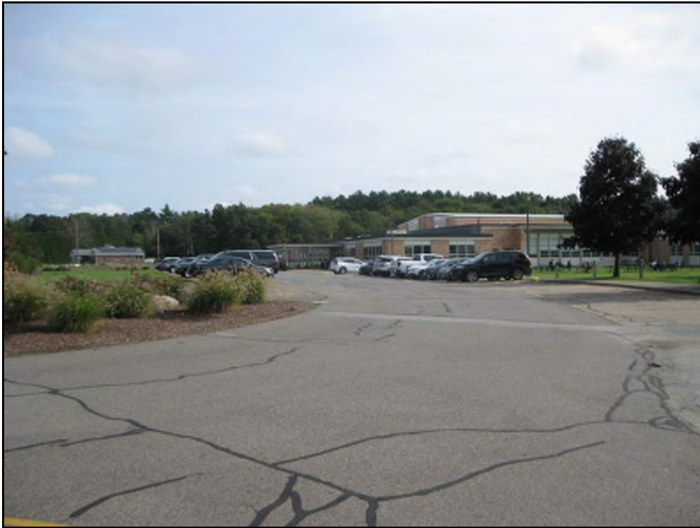
Northwest side of school
