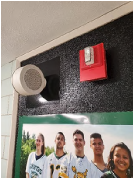
E9 – Typical fire alarm horn strobe
