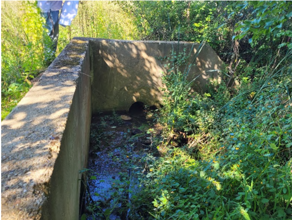
Figure 3: Concrete Headwall for 18-Inch and 30-Inch Outlet Pipes
