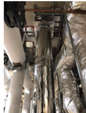
Photo 1- Boiler Venting
