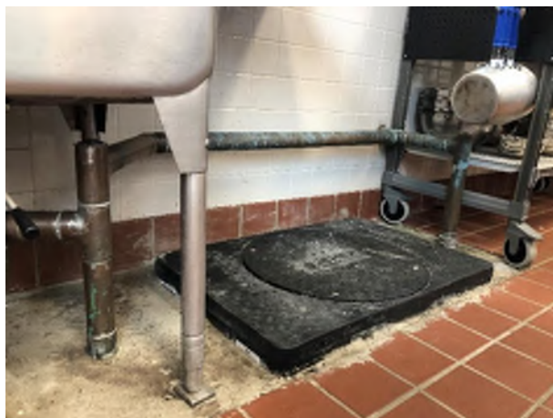
Recessed Grease Interceptor
