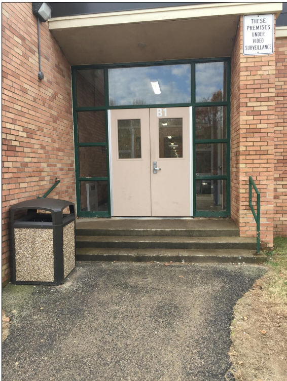
Main Student Entrance doors by student parking lot. Entrance is not considered accessible.
