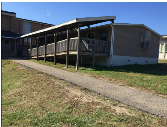
Modular classroom expansion with wood frame entrance stairs and ramp.
