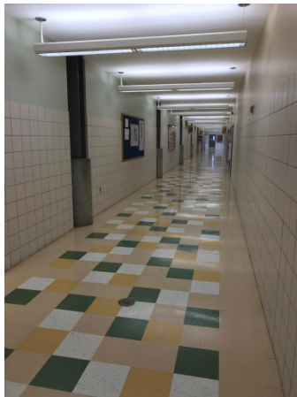
E19 – Addition Corridor
