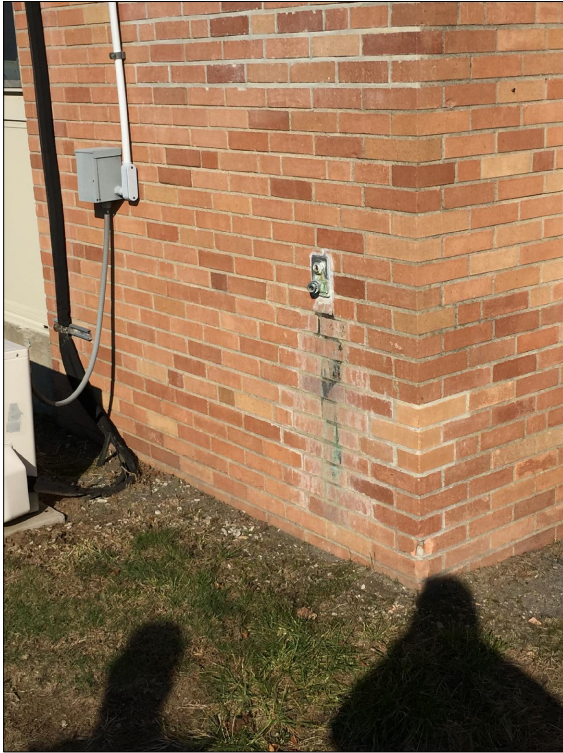
Typical exterior hose bib connection - masonry to repaired / patched.
