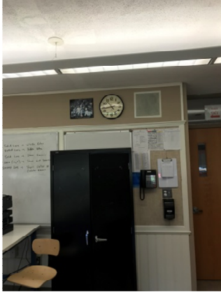
E21 – Typical Classroom Technology
