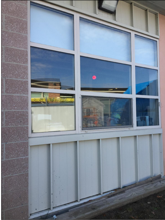
Typical window assembly at the 1992 addition - windows above with operable sections and metal wall panels below.
