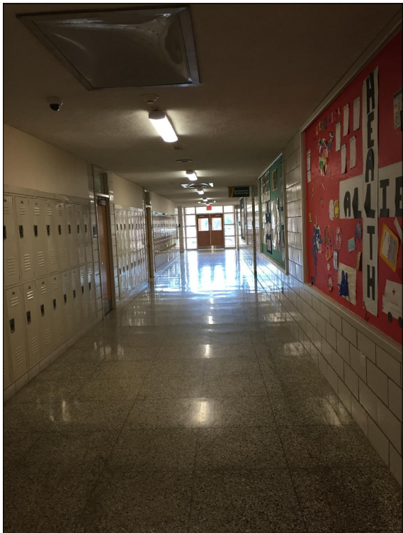
Typical corridor within the existing building. Finishes are typical - terrazzo flooring, glazed CMU block and plaster ceiling with skylights (some have been covered).
